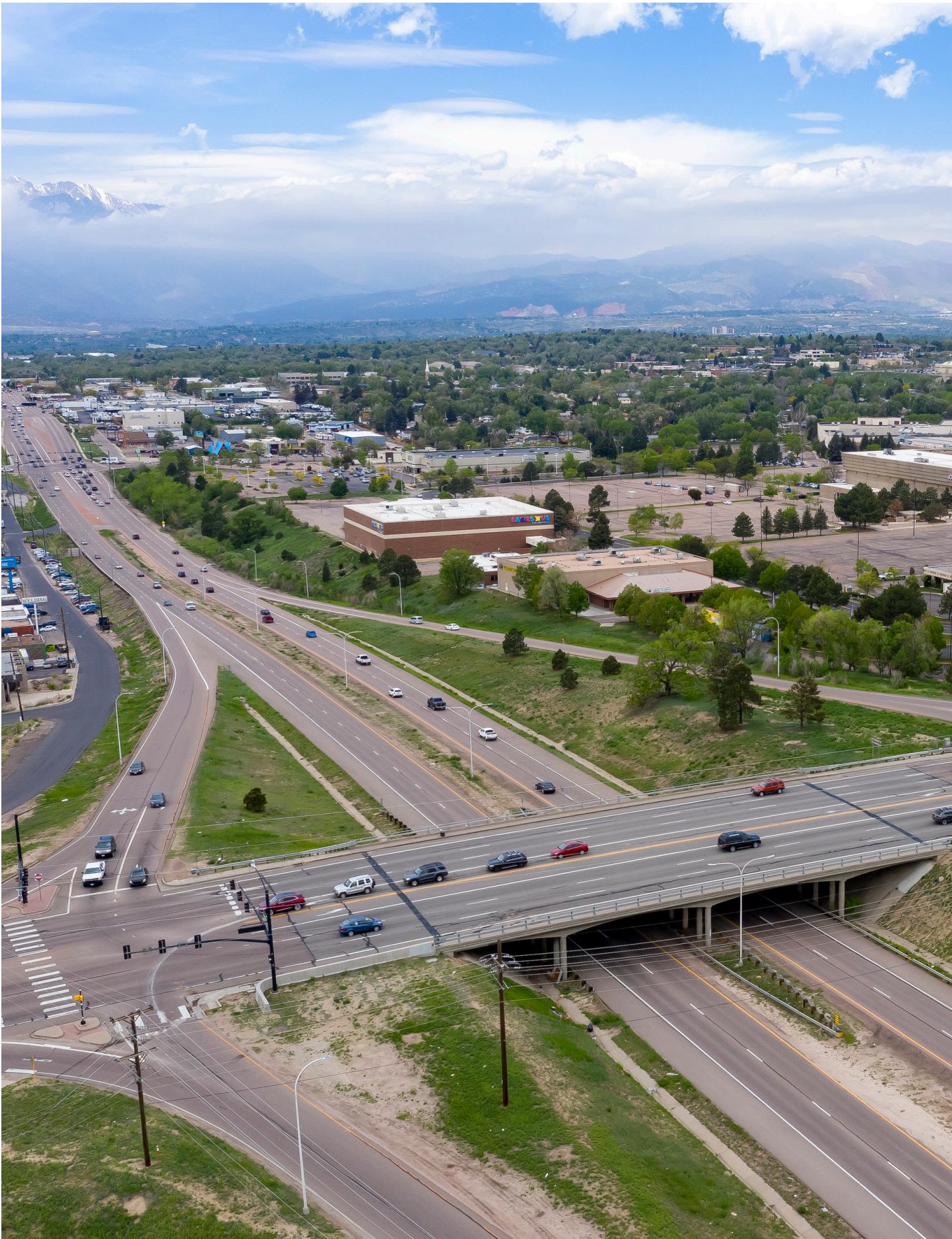
Photo Location: Platte Ave. and N. Academy Blvd.
